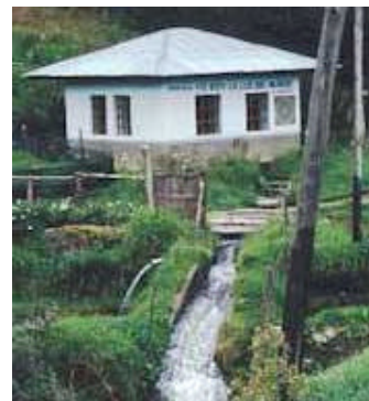
Community micro-hydro plant; Source: ITDG Peru.
